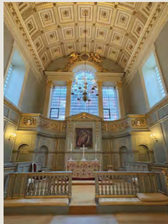
View East showing the elliptical barrel vault ceiling
