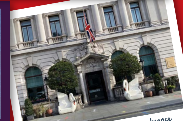
Sofitel Hotel, Waterloo Place entrance flanked by Royal Swan Sculpture seats
