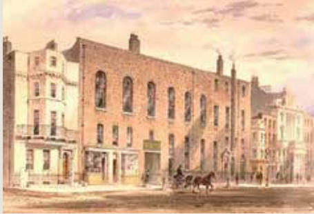
The Assembly Rooms, King Street looking west.
