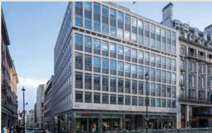
French Railways House, 180 Piccadilly and 48/50 Jermyn Street, for a proposed redevelopment on the right hand side of Duke Street, St. James's.
