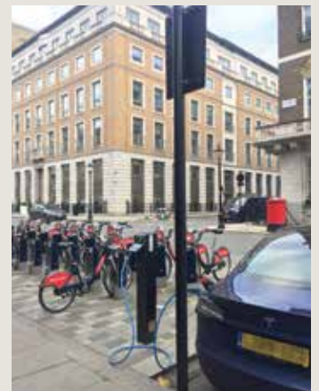
Recent, welcome electric car charging points, have however introduced trip hazards, with ill considered cable management.
