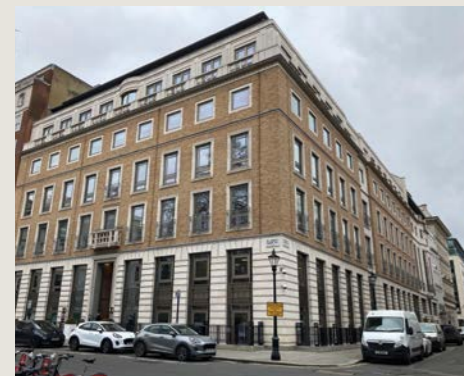
▲ Photo of existing building
