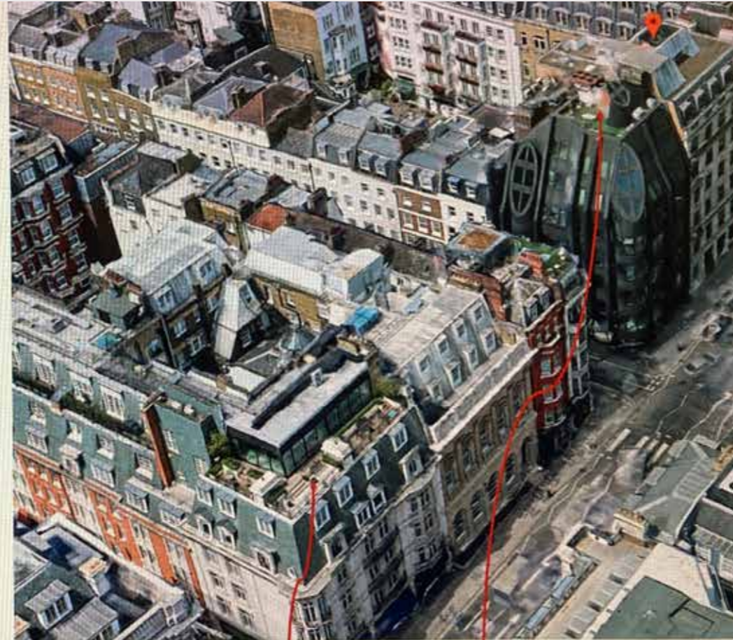
Roof Terrace at 72-73 St James Street
